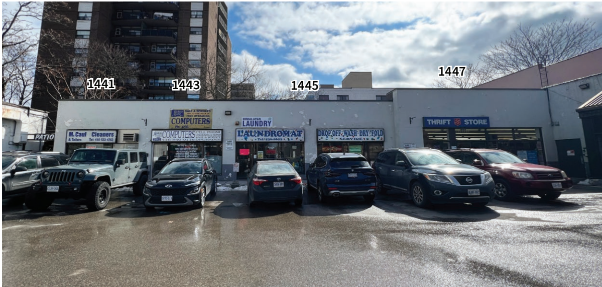
1441-1447 Queen Street West: principal (north) elevation. The entrance addresses are indicated above the building (ERA, March 2, 2023).
