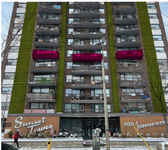
East elevation of 200 Jameson Avenue, located directly south of the Site, showing an example of the projecting balconies in pink (ERA, March 11, 2023).
