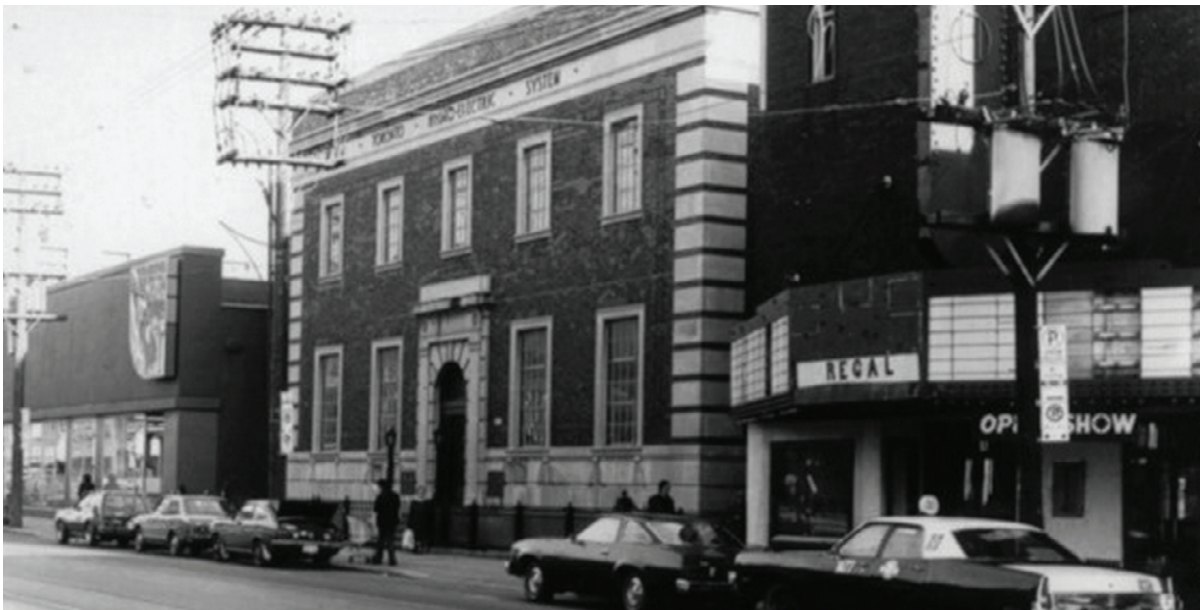
Undated photograph - Looking southeast on Queen Street West toward the completed Parkdale Substation (Sunnyside Historical Society).
