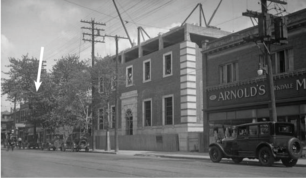
1927 photograph. Looking southeast on Queen Street West toward Jameson Avenue. The former buildings on the Site are indicated by a white arrow. The adjacent listed property 1457 Queen Street West (Parkdale Substation) under construction is at centre (City of Toronto Archives; annotated by ERA).
