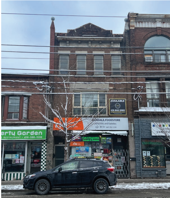
Principal (south) elevation of 1506 Queen Street West (ERA, March 11, 2023).
