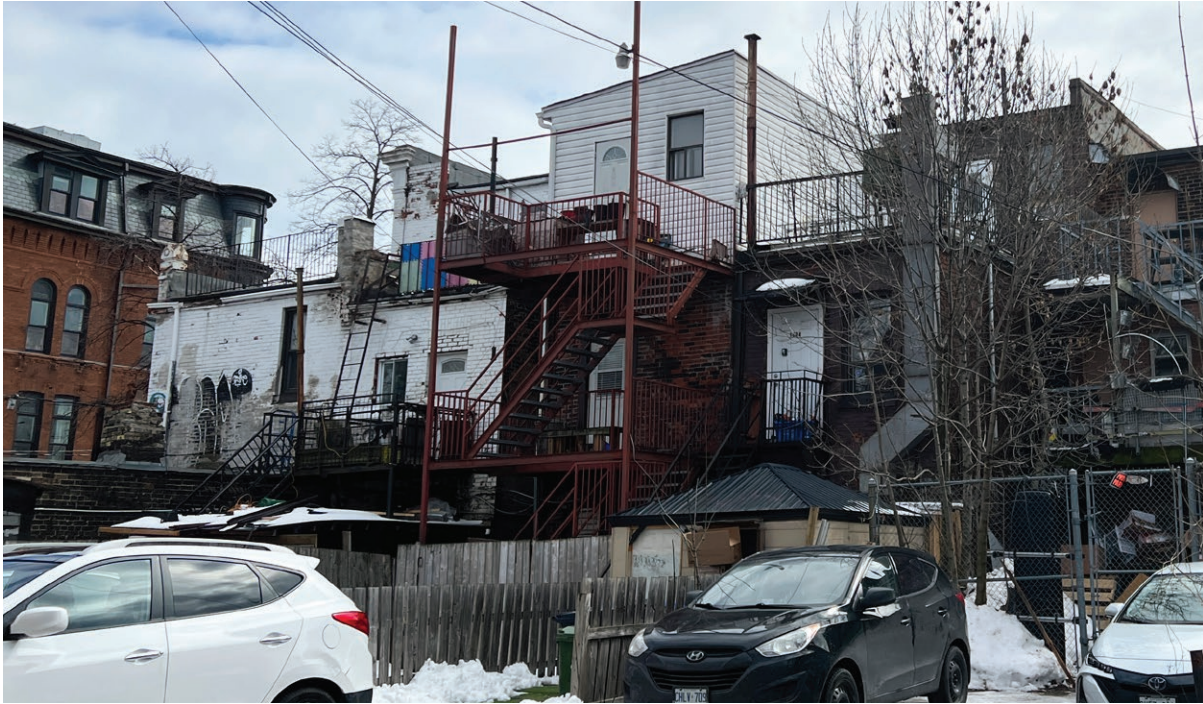
Rear (north) elevation of 1498-1504 Queen Street West (ERA, March 2, 2023).
