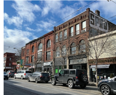
Historic main street character on Queen Street West, west of O’Hara Avenue (ERA, March 2, 2023).
