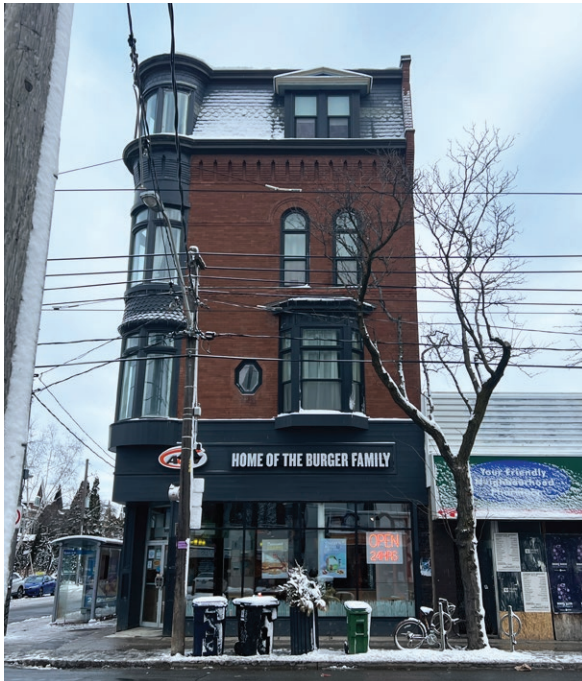
Principal (south) elevation of 1496 Queen Street West (ERA, March 11, 2023).
