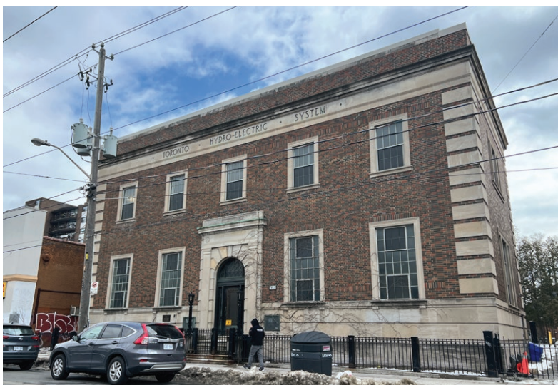
Parkdale Substation Toronto Hydro-Electric Commission building located at 1457 Queen Street West (ERA, March 2, 2023).
