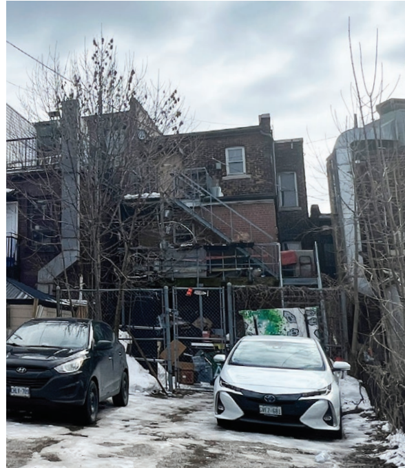
Rear (north) elevation of 1506 Queen Street West (ERA, March 2, 2023).
