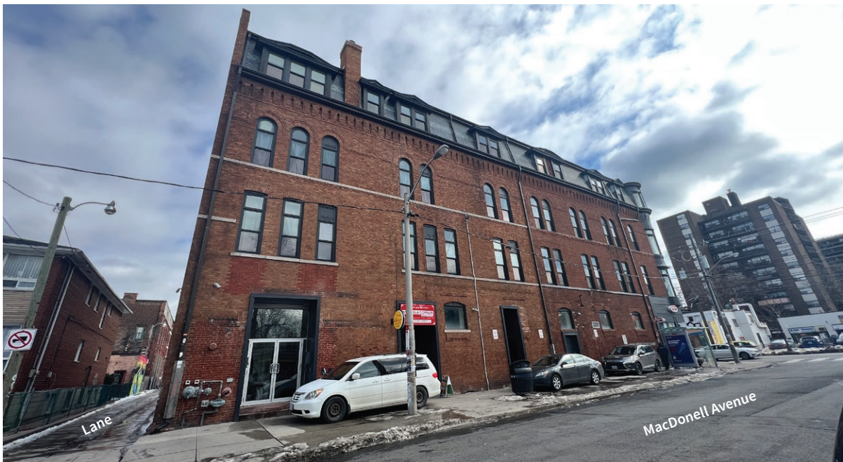
West elevation of 1498-1504 Queen Street West (ERA, March 2, 2023).
