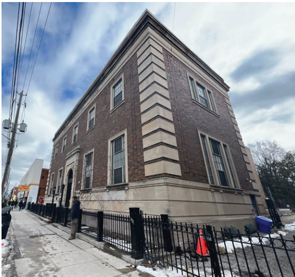
West elevation of 1457 Queen Street West (ERA, March 2, 2023).
