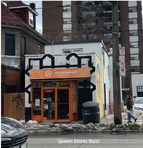
1439 Queen Street West: principal (north) and west elevation (ERA, March 2, 2023).
