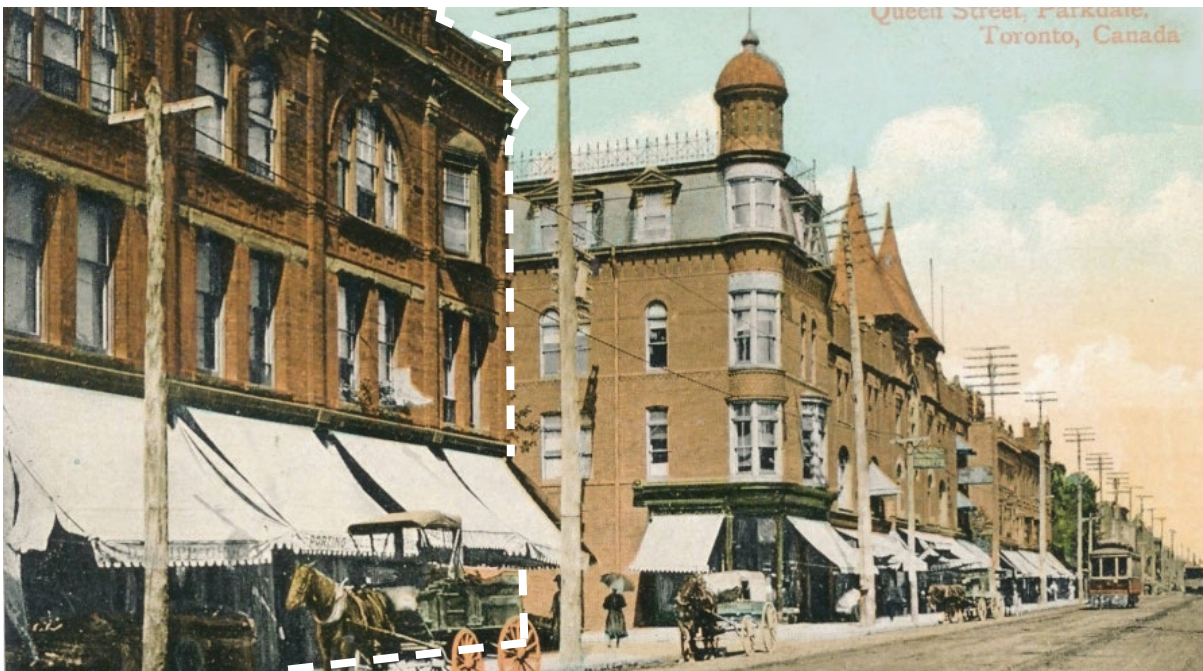
Undated postcard looking east on Queen Street West, past MacDonell Avenue. The property at 1498-1504 Queen Street West is outlined in a white dashed line (City of Toronto Archives; annotated by ERA)
