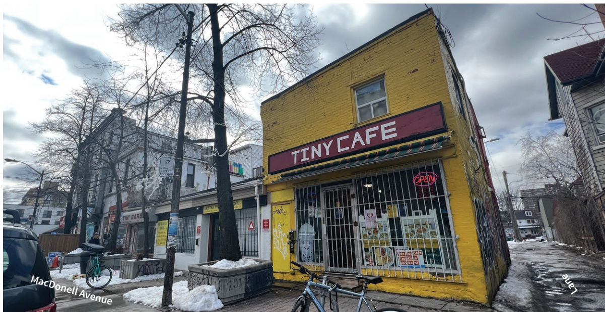
Principal (east) elevation of 1498 Queen Street West and 2-10 Laxton Avenue (ERA, March 11, 2023).
