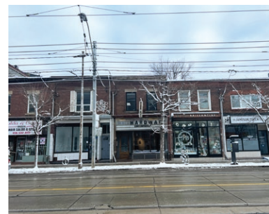
Fine-grain main street commercial buildings at 1518-1524 Queen Street West (ERA, March 2, 2023).
