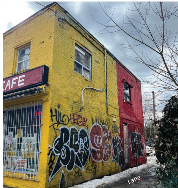
Rear (north) elevation of 10 Laxton Avenue (ERA, March 2, 2023).
