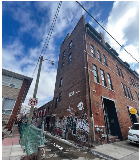
Rear (north) elevation of 1496 Queen Street West (ERA, March 2, 2023).
