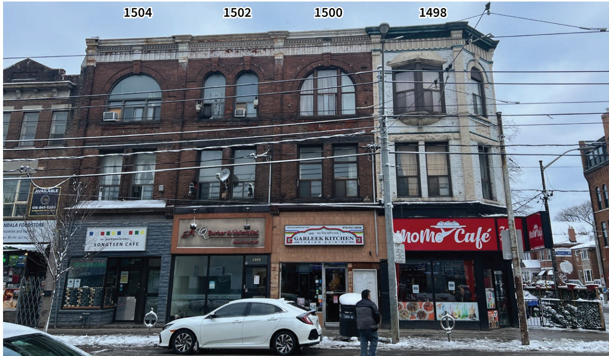
Principal (south) elevation of 1498-1504 Queen Street West (ERA, March 11, 2023).
