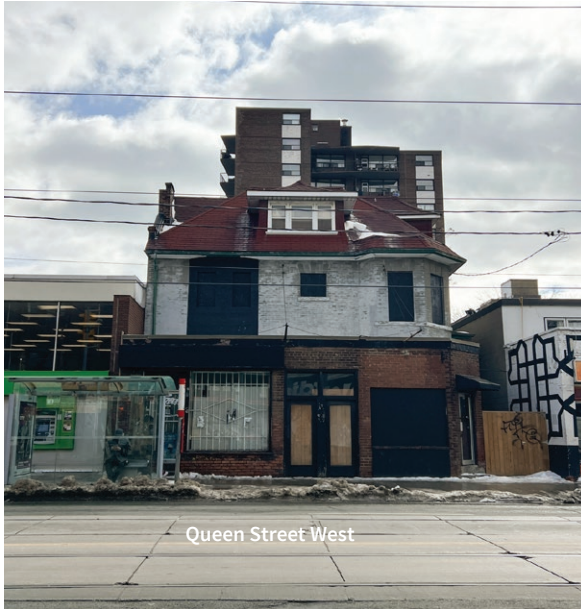
1437 Queen Street West: principal (north) elevation (ERA, March 2, 2023).
