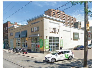
Medium-scale commercial building at 1357 Queen Street West (Google Earth, 2021).
